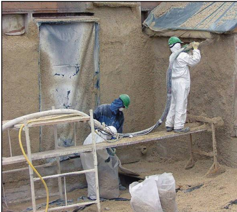
FIGURE 7.32 Spray application of hemp–lime composite to a building. Photo courtesy of Steve Alin.
