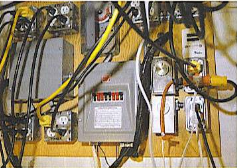
If you must wire your own grow room electricity, make sure to plan ahead of time. Attach junction boxes, timers, etc., to a board, and mount the board on the wall once the appliances are in place.
