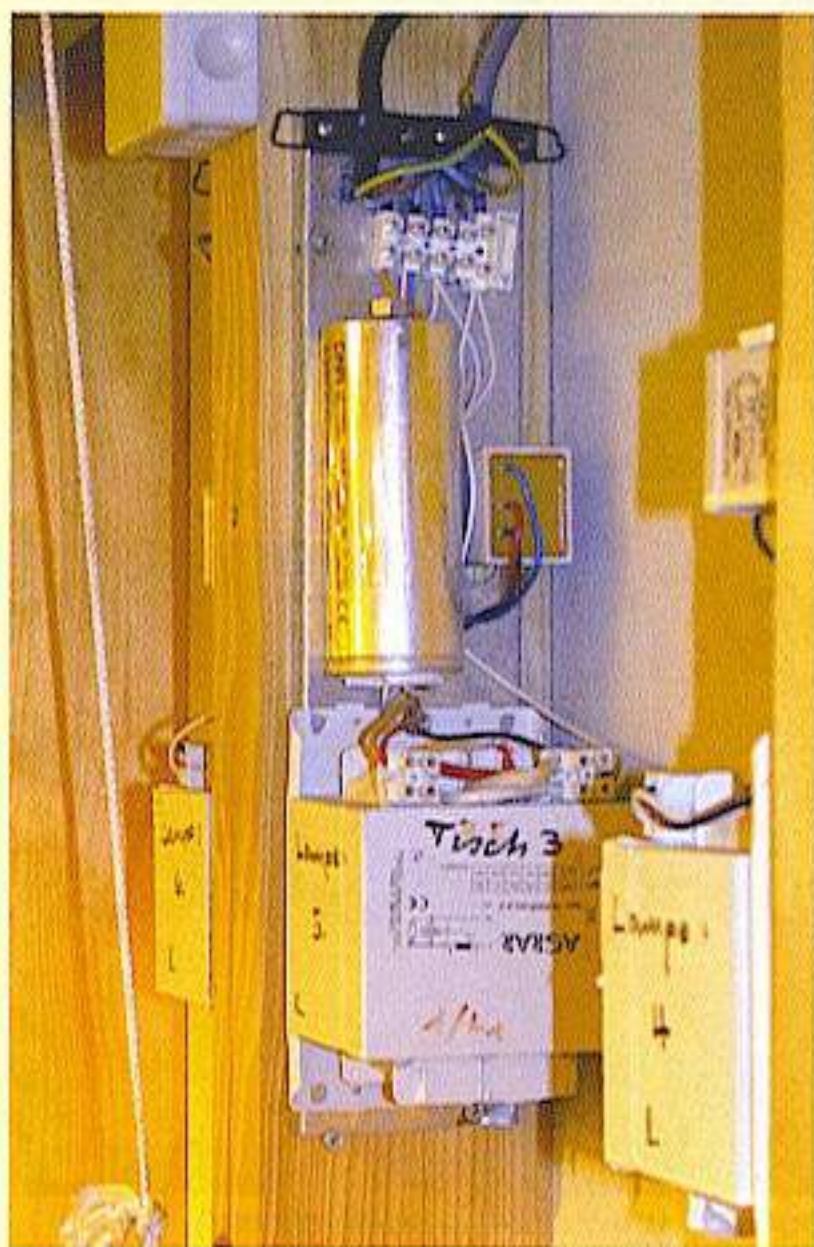
Attach ballasts to the wall so they are out of the way in the garden.
