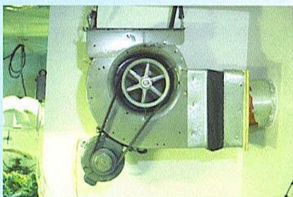
This fan is suspended by bungee cords to shunt noisy vibrations. Always keep your fans well lubricated so they run smoothly and quietly.
