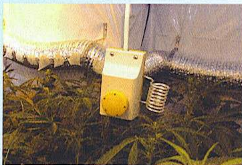
To control the air temperature, hang the thermostat near the canopy of the garden.
