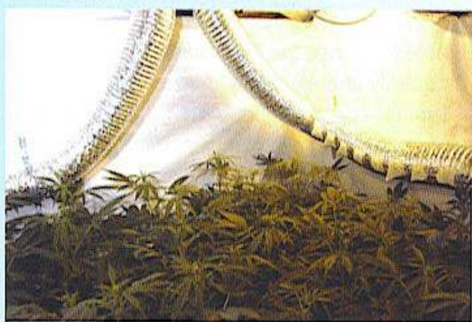
Intake air ducting has holes covered with duct tape. Air flow is directed by removing pieces of tape.
