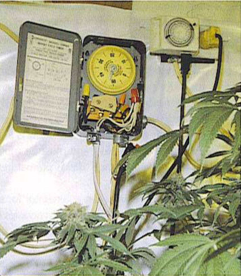
The mechanical timer on the left will operate several lamps at the same time. The digital timer on the right operates a single 1000-watt HID.
