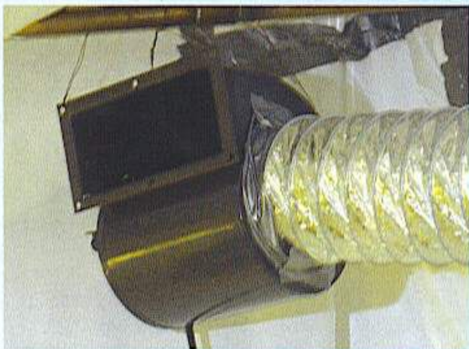
This blower is at the end of intake air ducting. The main fan is at the other end.
