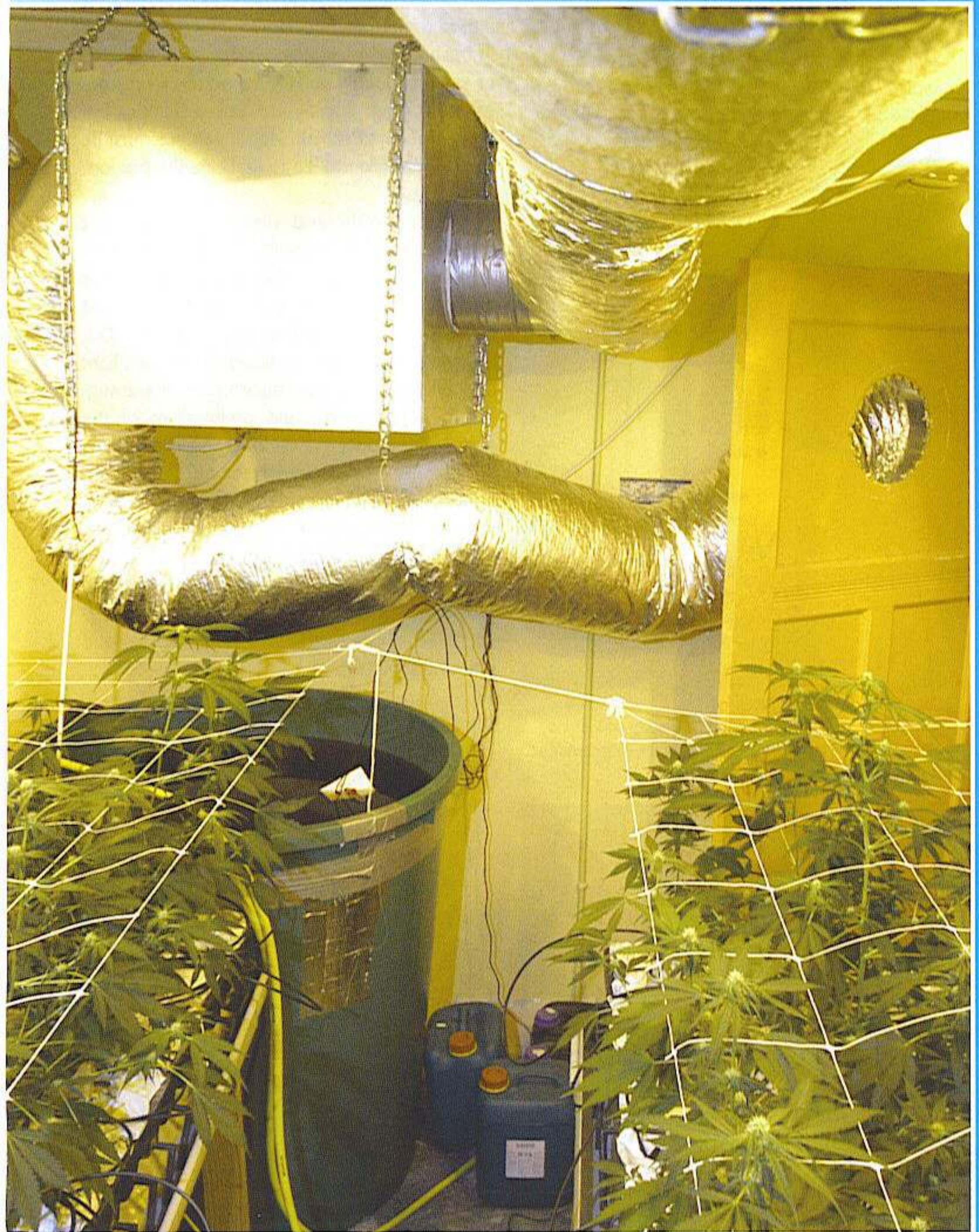
A carbon filter and ozone exchange box dominate the landscape in this Dutch grow room.
