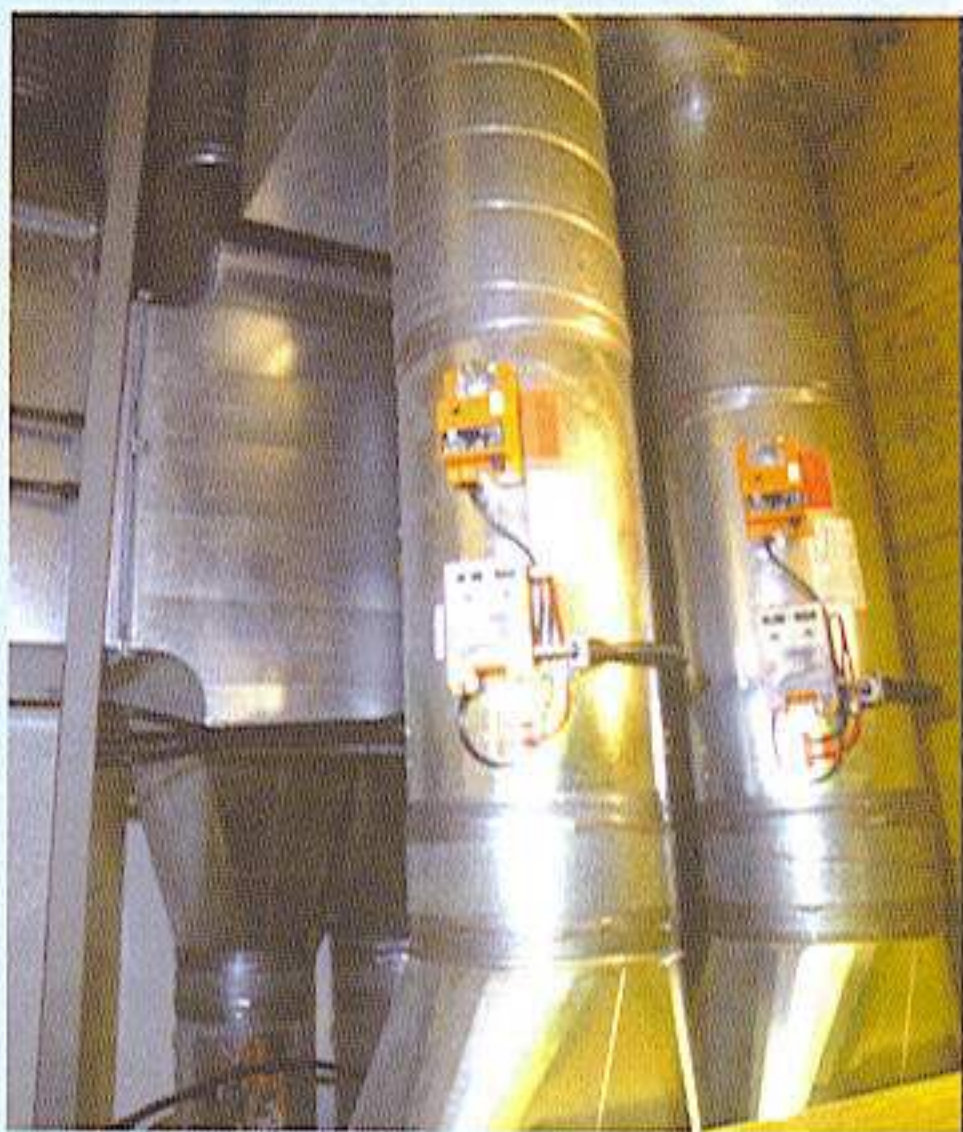
Ozone generators are located inside ducting. Grow room air mixes with ozone in ducting and big metal box. Air smells fresh and clean once treated properly with ozone.
