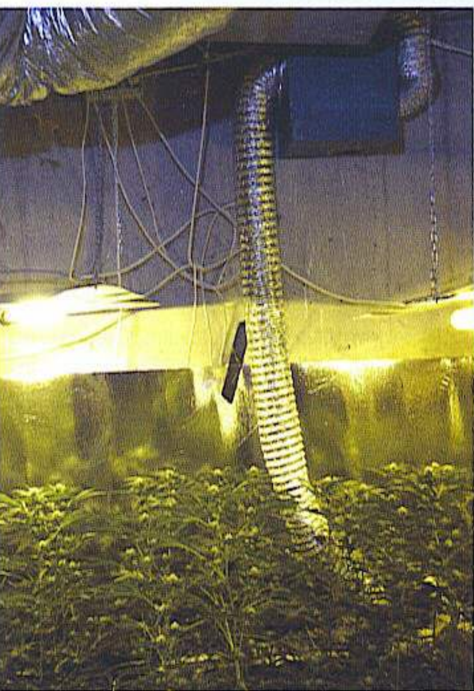
A booster fan in the gray box pushes intake air down the duct to the bottom of the garden.
